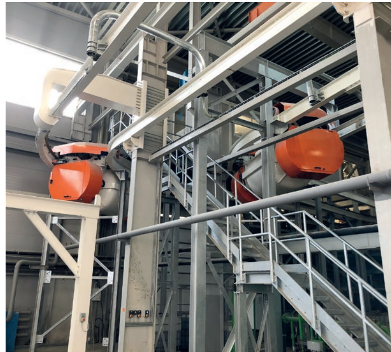
Precast plant integration
